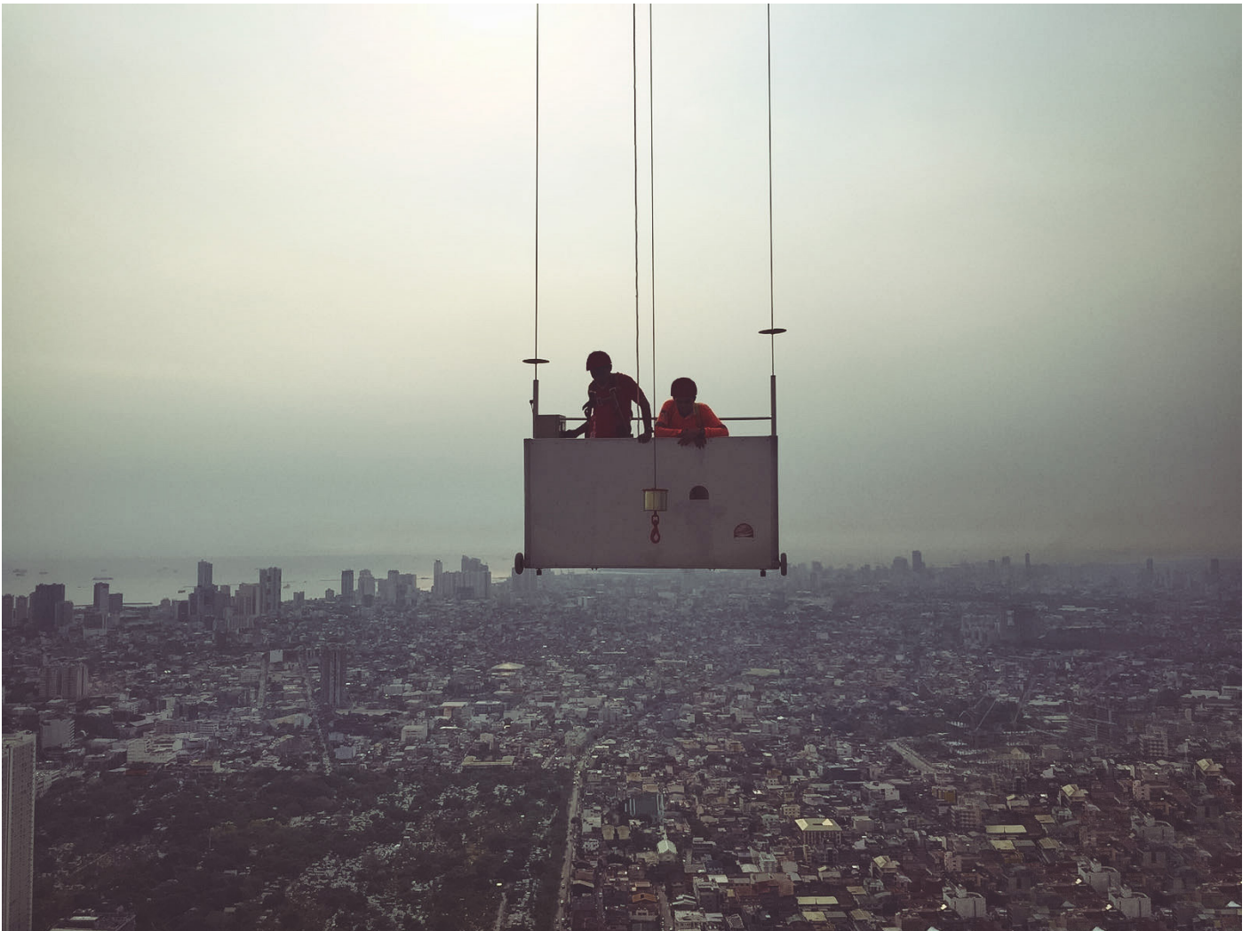
Cradle for two users and auxiliary material hoist of 400 kg.
