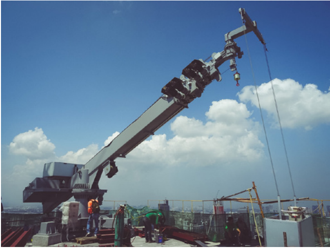
BMU Type S with telescopic jib of 20,5m reach.
