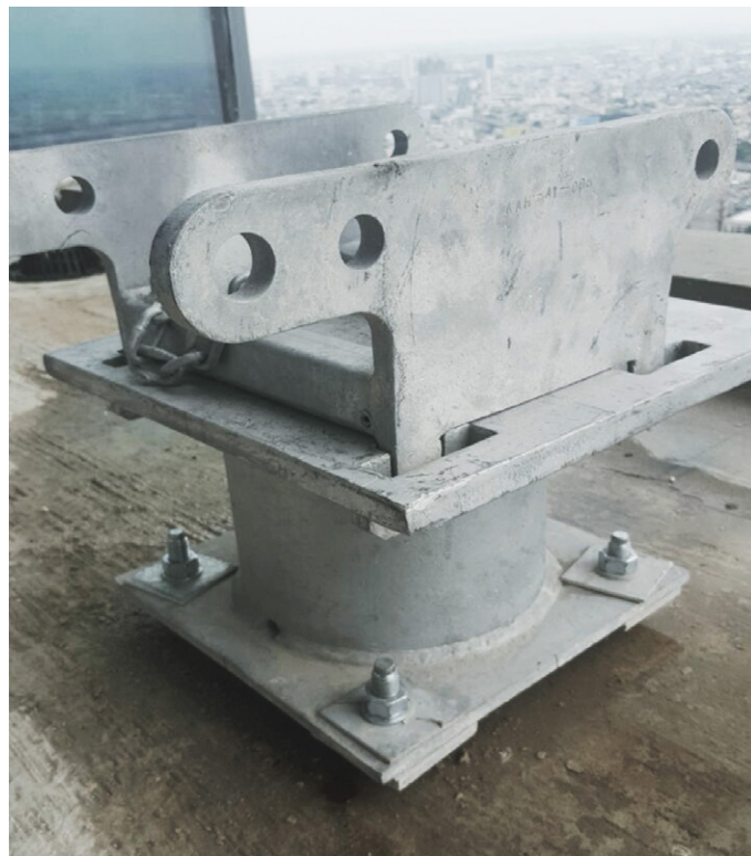
Fixed base for temporary davits.
