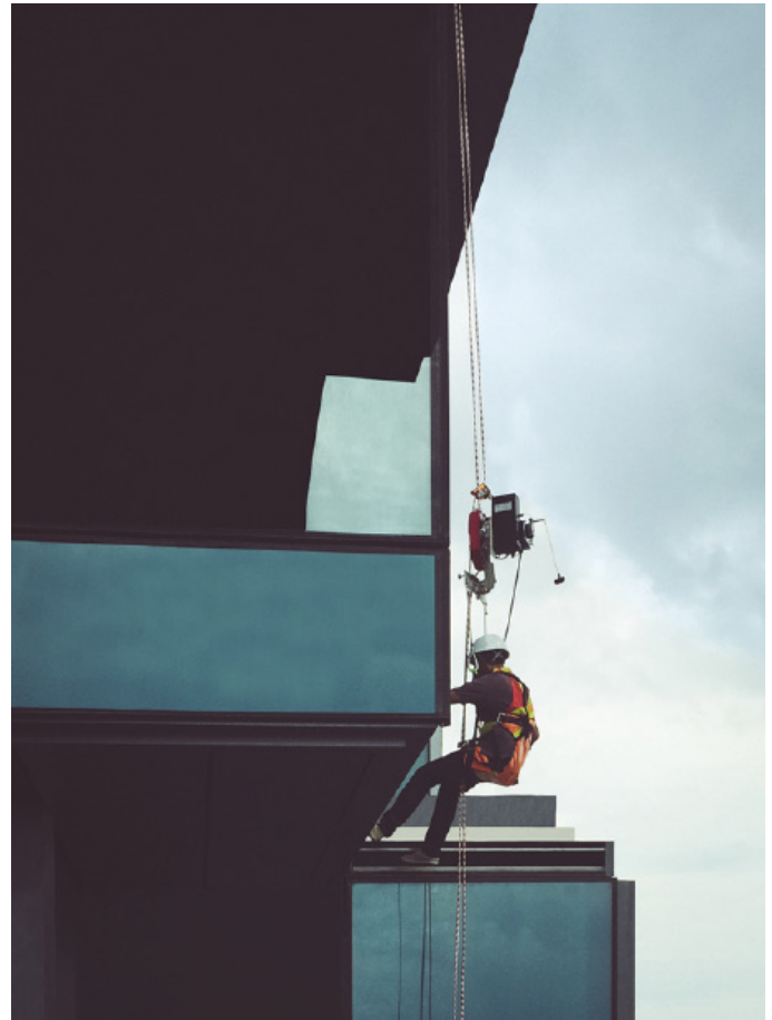
RopeClimber man-riding autonomous hoist suspended on Davit system.
