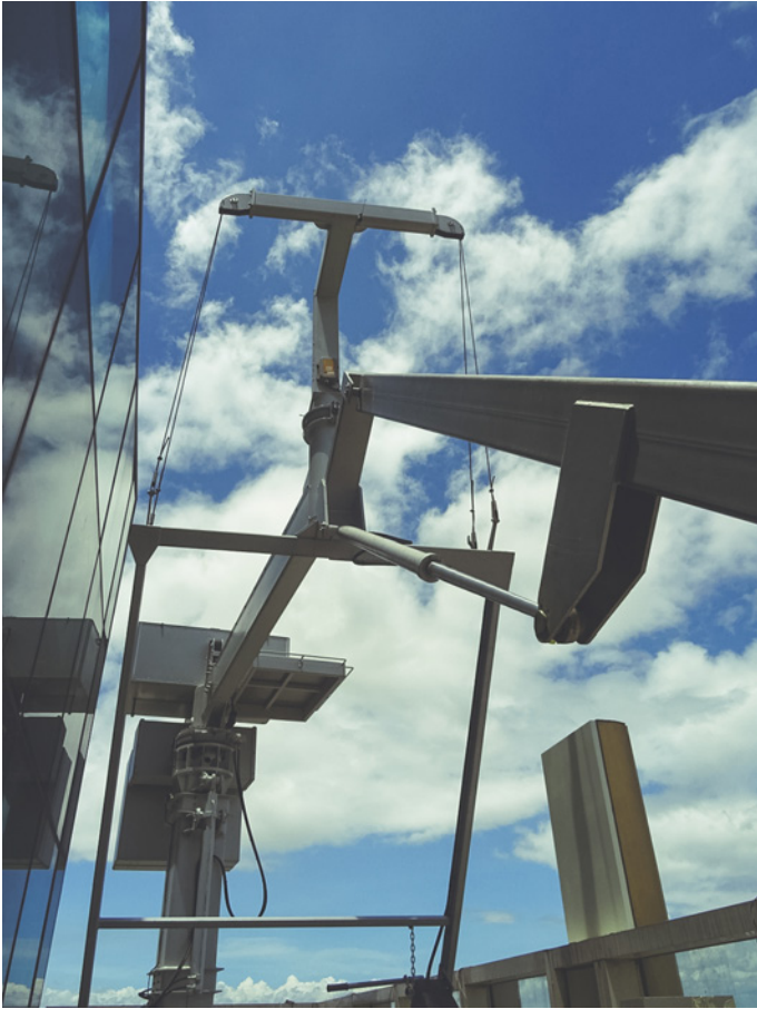
Pantograph system to reach the concealed facade.
