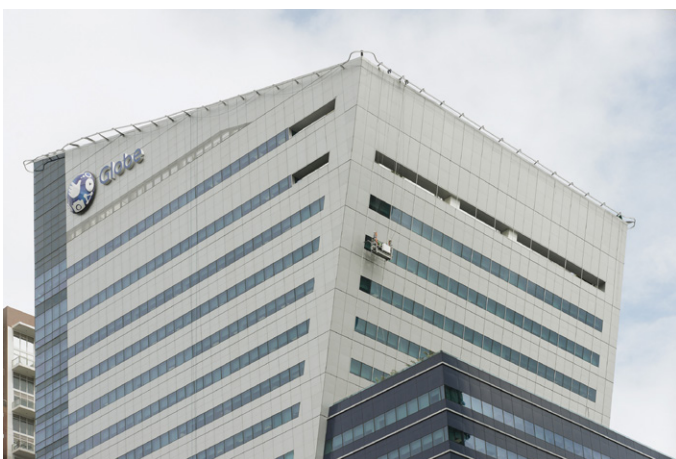
Climbing SafeAccess rail with cradle suspended.
