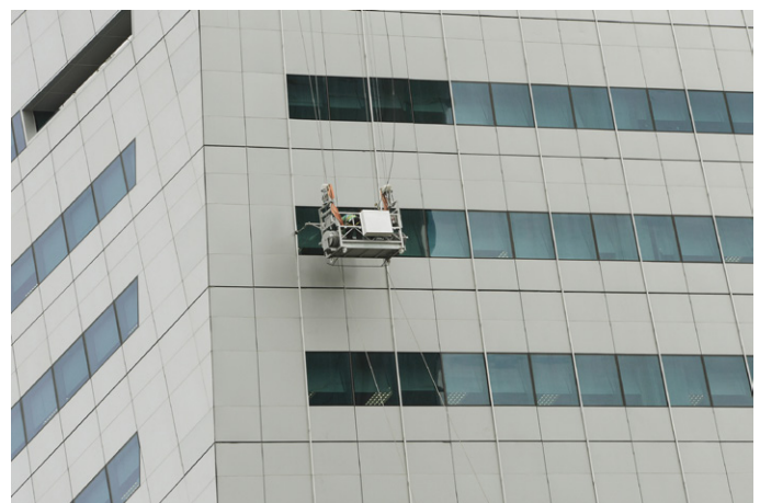
SecuRail as restraint system for the cradle.
