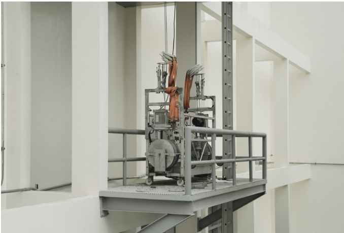
Cradle to courtyard maintenance.
