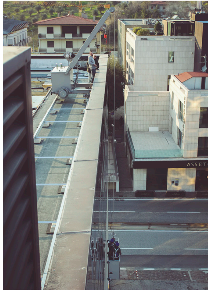
The counterweight system is the machine's chassis itself.
