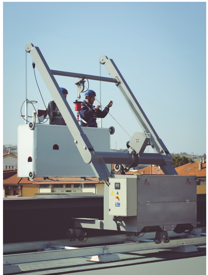
BMU FBA Type 2: a standard machine.
