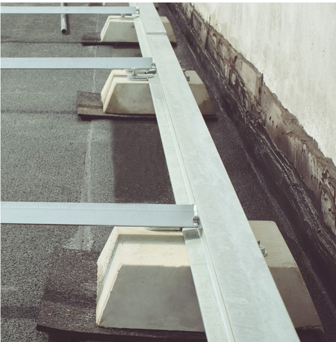
Concrete dice to support the rail without penetrating the membrane roof.
