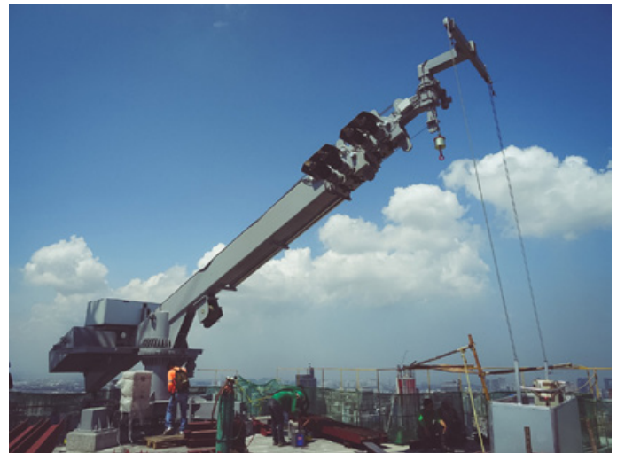
Trump Tower: a compact FBA S machine stationary and through slewing all facades can be reached confortably. Installed in Manila, Philippines.
