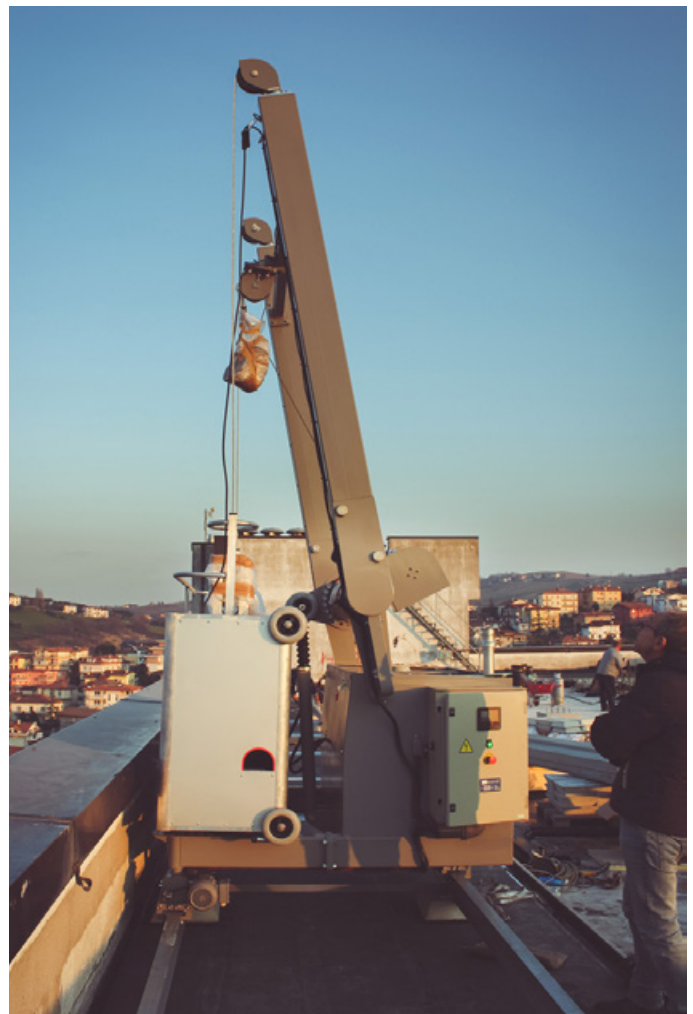
FBA 2 in parking position, just after its installation.
