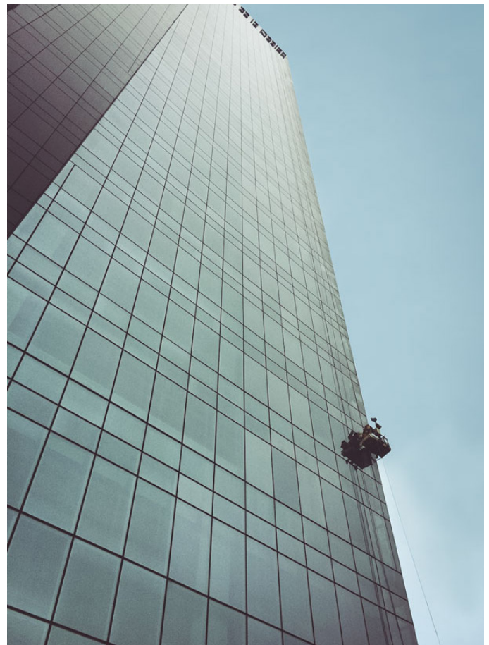
Cradle suspended from BMU type FBA 40.
