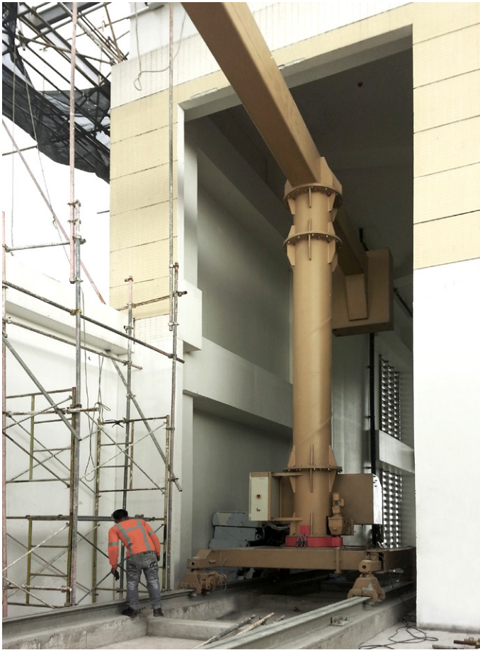
4 meter mast to overpass the parapet.
