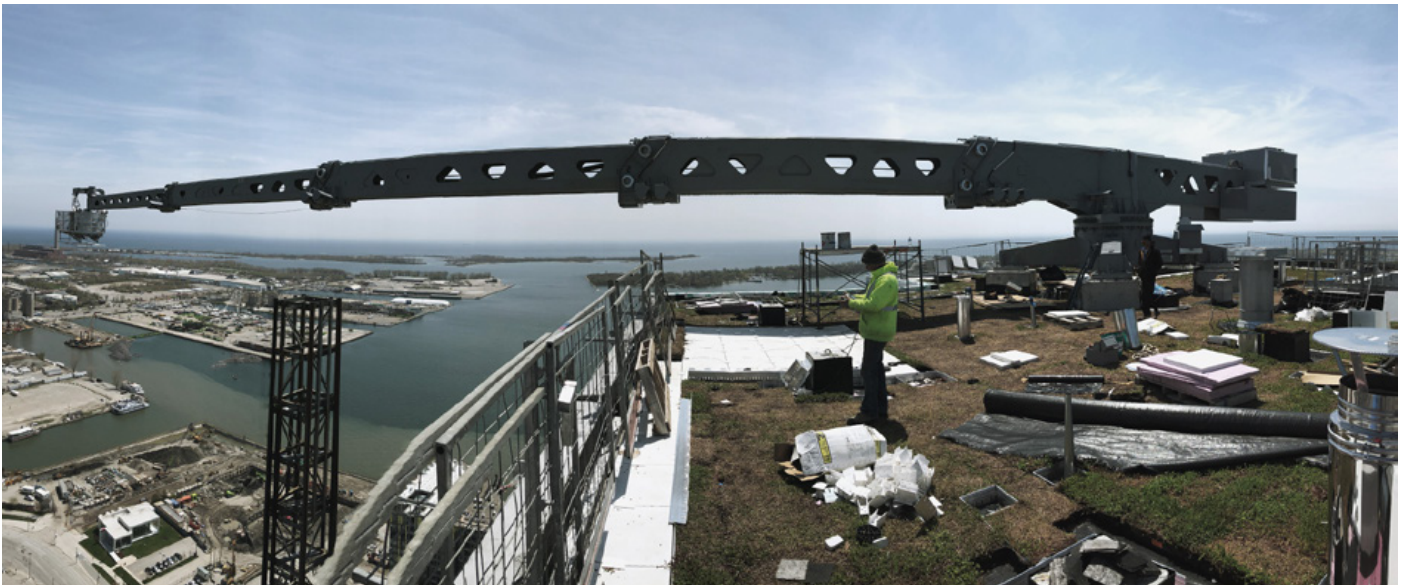
A special multi-layer lifting hoist equipped with 6 steel ropes to suspend the 3-module layer from a height of 226m.
