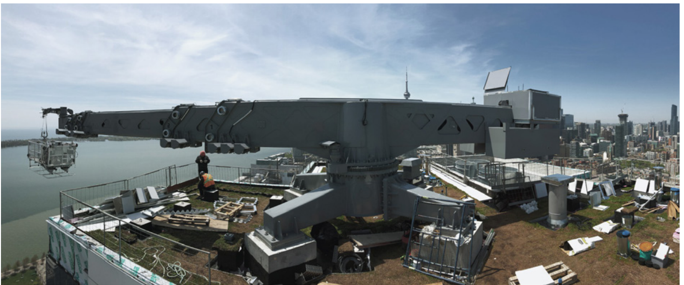
The BMU telescopic arm a) displayed at its maximum outreach of 36m and b) retracted.
