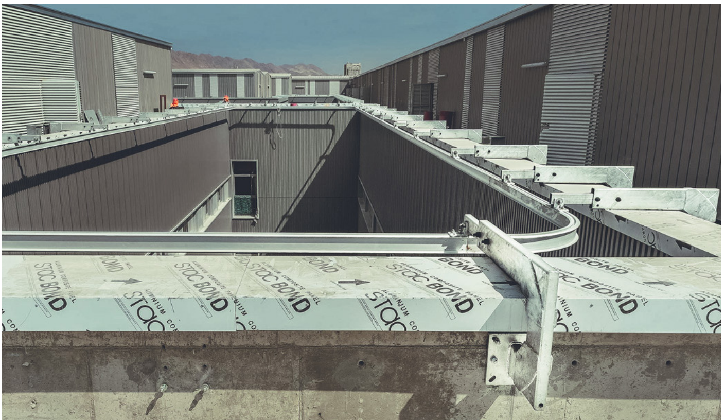
SafeAccess monorail fixed to the inner parapet. The brackets have been designed according to SIRVE's antisismic parameters.
