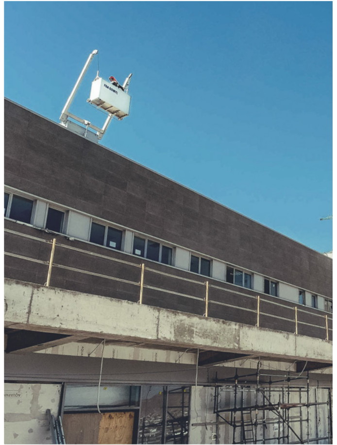
BMU Type FBA 2. The lightest solution with two jibs that allows working positions with different reaches and a parking position for the cradle.
