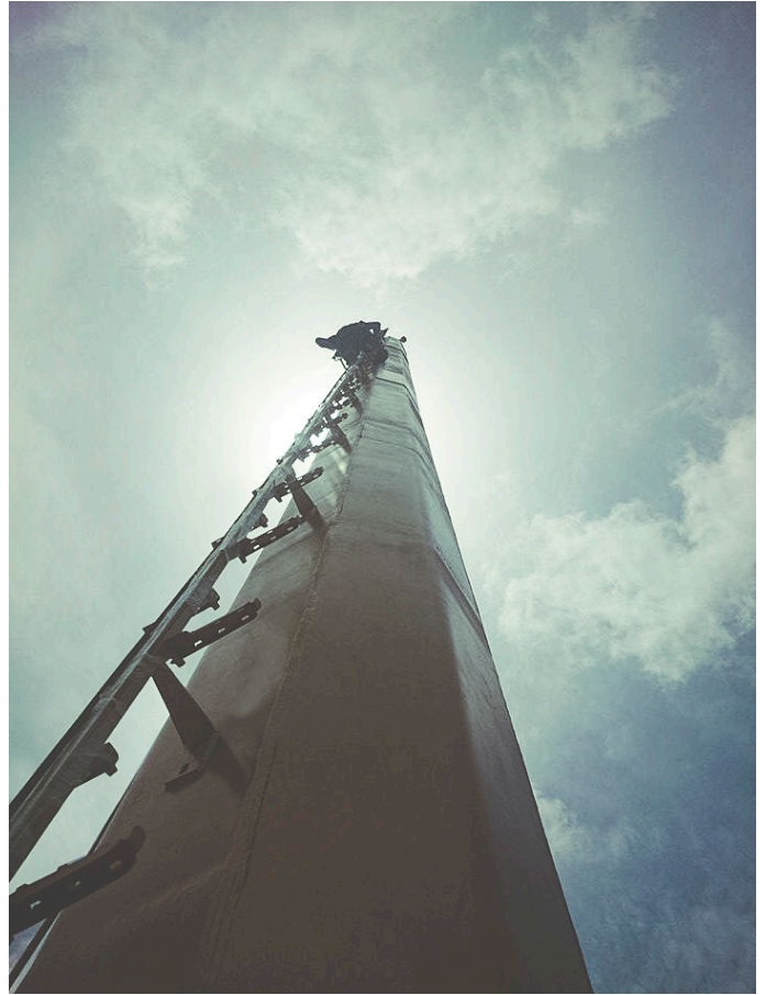
SecuRail ladder for the spire antenna maintenance.
