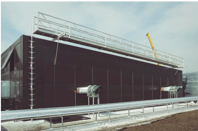
Horizontal traversing gantry designed to clean a fragile roof deck.
