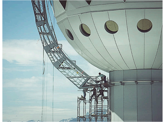
Gantry designed to cover a fully spherical construction.
