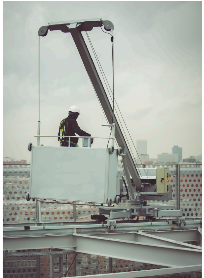
BMU FBA 1 installed in Spain. The rails are fixed to an upper structure behind a 3m high parapet. The machine has a jib luffing, in order to pass the cradle over the parapet.
